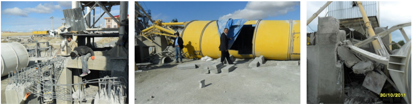
a. Supporting concrete failure [14] b. Collapse due to brittle welded connection failure [14] c. Local buckling and anchorage failure [14]
