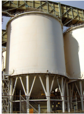
b. 10,000 ton steel grain storage, Australia [2]
