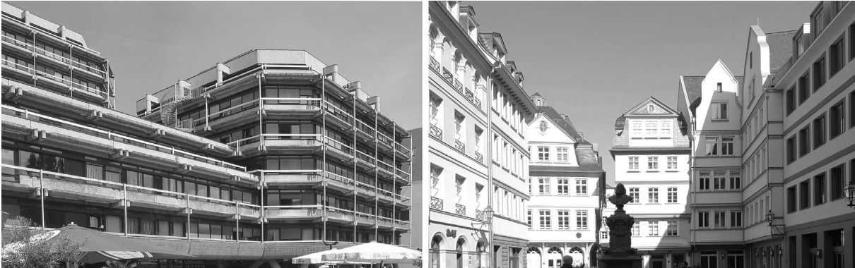
Fig. 3 - Frankfurt am Main, Dom Roemer Areal: Technical Townhall (1972-74) / reconstructed Hühnermarkt (Source: Wikipedia / Caja)
