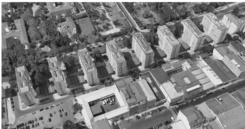
Fig. 6 Aerial view of the buildings along the avenue, seen from the South. Photo: Google, 2018. Architect: Jorge Segurado, 1958. We can see the modernist effect of the sequential volumes to be perceived from the traffic along the avenue. The housing blocks are connected by one-floor commercial buildings, recessed from the avenue and therefore creating small squares and gardens for public use.
