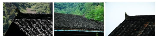
Figure 21. The Lifted with Tile Stacks.
