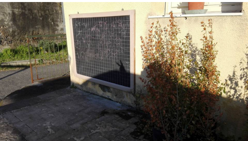
Fig. 9- One of the school of the comprehensive institute Giovanni XXIII, the Santa Maria delle Grazie School in Acireale, Sicily that evokes an open classroom space thanks to the presence of an outdoor blackboard 11
