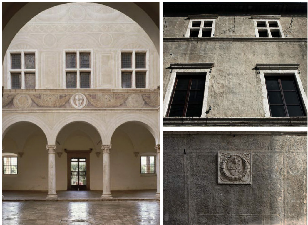
Fig. 4. Pienza, Piccolomini and Ammannati palaces, detail of graffiti (photos by the authors).
