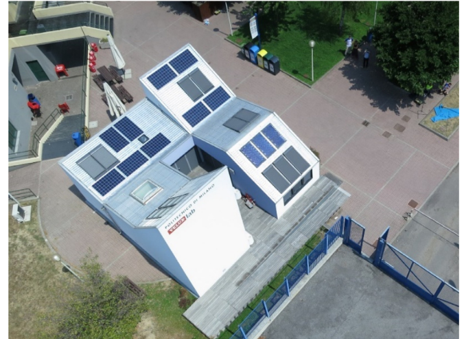
Fig. 19. Aerial view of the VELUXlab, with photovoltaic and solar panels systems installed on the pitched roof.
