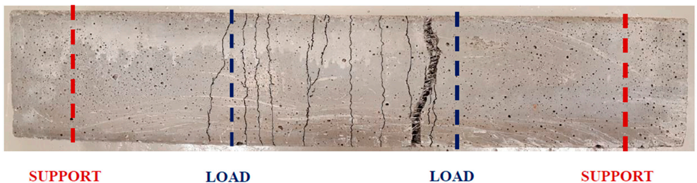
Figure 2. Typical final crack pattern observed on the bottom surface after 4-point bending test.
