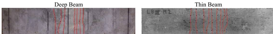
Fig. 6. Typical crack patterns after pre-cracking for deep beams (a) and thin beams (b).
