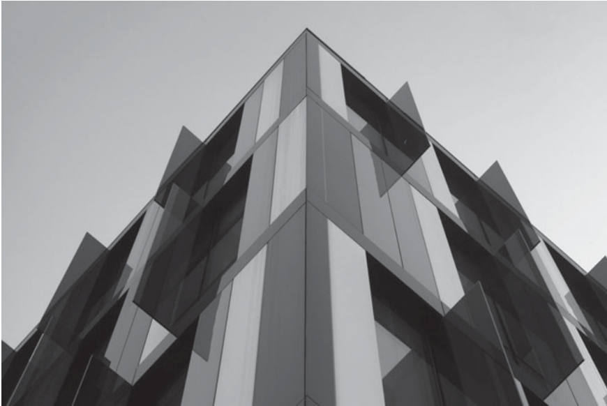
Fig. 8.14 Interactive surfaces as “mediatic skins” according to the development of criteria of “hypermediate perception” and to the inclusion and dilution of visual transitions. Gianandrea Barreca and Giovanni La Varra, RCS Media Group Headquarters, “B5” Building, Milan © Courtesy of Focchi S.p.A.
