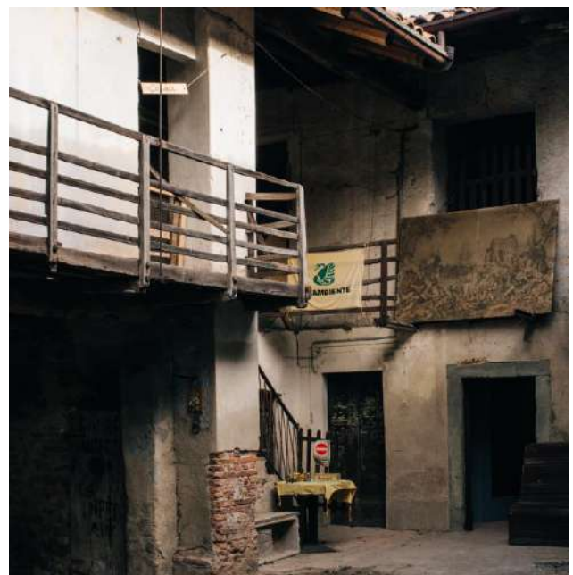
Fig. 3: The entrance of Casamatta
