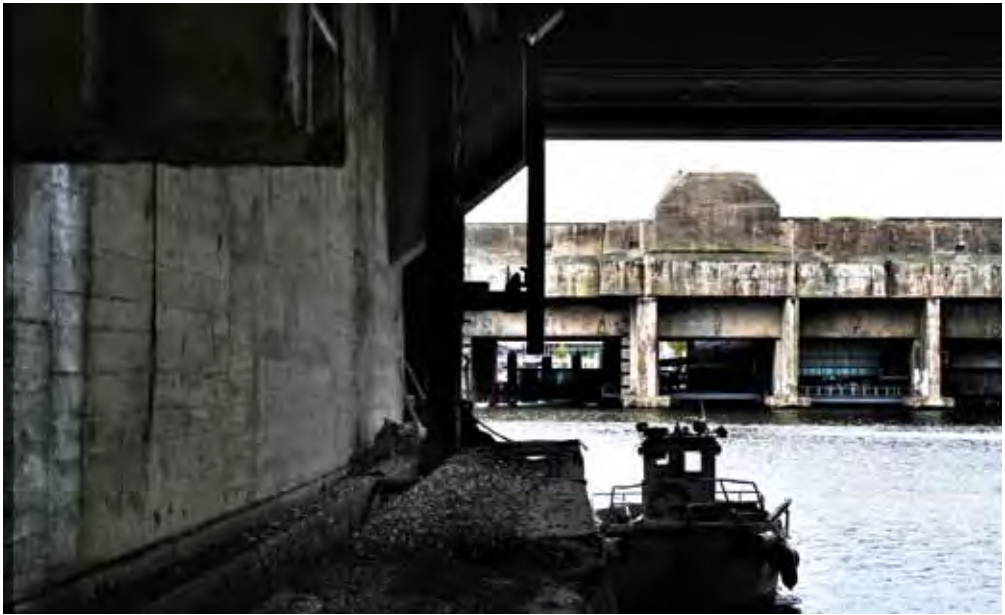
View of one of the interior gateways through the corridors of the bunker. Saint Nazaire (Ph. Claudia Brunelli)
