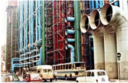
Renzo Piano, Richard Rogers, Centre Pompidou, Parigi, 1972-77 / Renzo Piano, Richard Rogers, Centre Pompidou, Paris, 1972-77.
