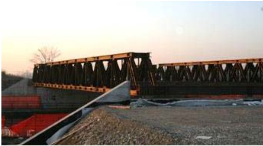
Figure 2. Overview of the bridge structure during the construction works.
