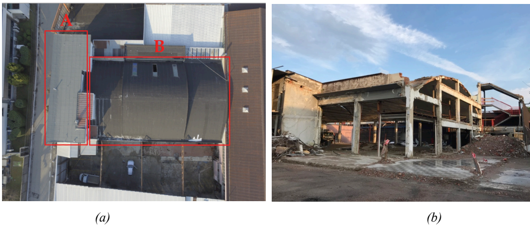
Figure 3 – Warehouse object of the analysis
