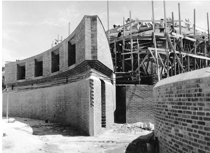
Figure 7. One of the pendentives of the dance pavilions' domes during construction. As can be noticed, the tiled intrados of the pendentive was configured as a work form for the subsequent concrete casting (ISA archive).
