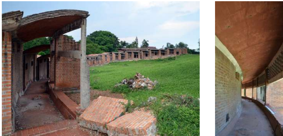
Figure 24. The cracks running along the crown of the vaults covering the upper corridor of the gusano building (photo by the authors).
