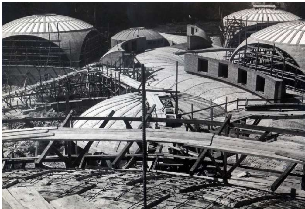
Figure 12. The reinforcing steel net positioned above the ribbed cap of the choreography theater before the second concrete casting (ISA archive).
