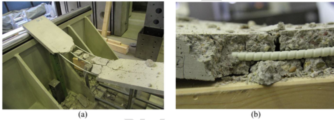
Fig. 16. Slab V10 – damage at failure: (a) slab at testing setup, (b) detail of embedded reinforcing bar (photo courtesy of authors [43]).
