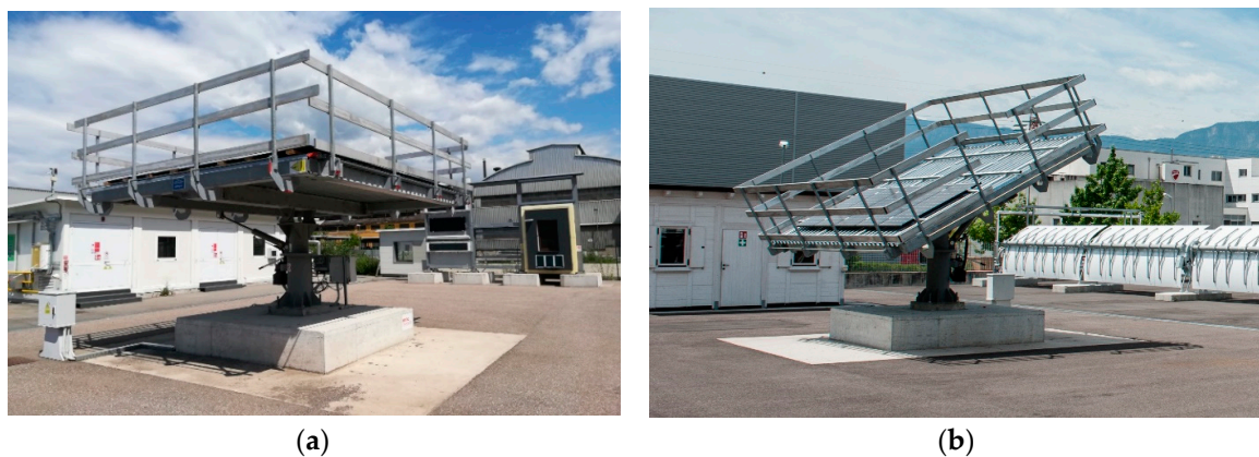
Figure 2. Outdoor PV integration lab: (a) view of roof in horizontal configuration and façade testbeds; and (b) detail of rotating configuration of the of the roof testbed.
