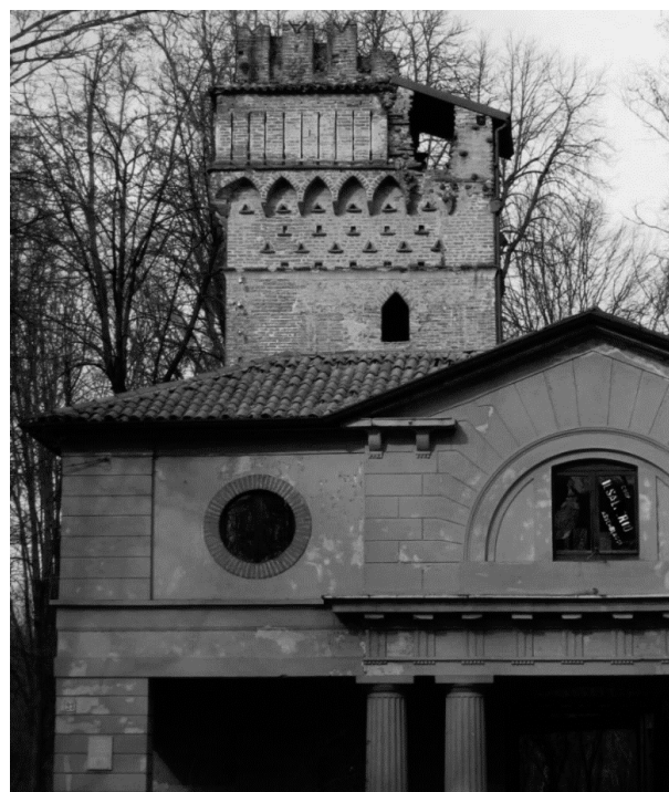
Figure 5. Detail of the main façade.
