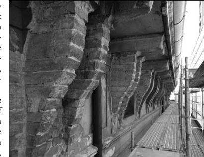
128. The semi-volutes of the cornice were formed with 15 courses of bricks. A couple of bricks placed on edge above the eighth course give resistance to the section, compensating for the forces of momentum and shearing stress at the point in which they are at a maximum. This skill is present in the first fifteen semi-volutes from the eastern end of the façade, facing in the rest towards the west and signalling a return to construction work and confirming how the renovation work and raising of the domus magna and of Ferrante Magio's house, including the cornice and the eaves, anticipated the corresponding alterations of casa Lotica which were completed before 1692 when the interiors had not yet been finished.
