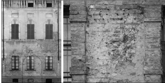
133. Ten bricks placed head to head illustrate the location of a semi-circular arch, between the third and fourth windows on the ground floor. Extending the arch illustrated by the bricks, the shape of a barrel vault can be seen with a width of a little less than 3.8 metres and 5.3 metres high, equal to approximately 7 x 11 Cremonese "braccia", corresponding to the passageway of the house belonging to Ferrante Magio.
