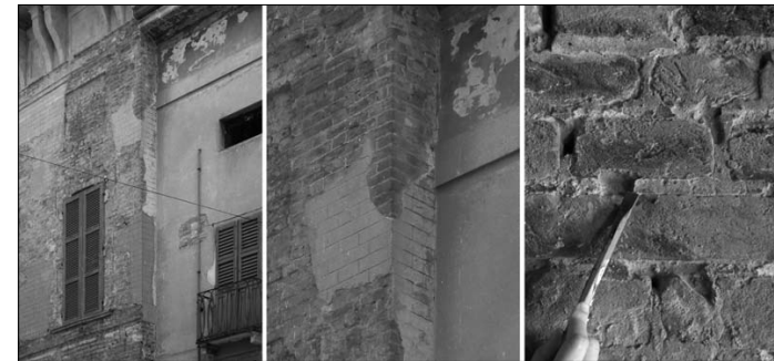
126. Corresponding to the western edge, the brickwork of the façade turned back to divide the adjacent lots. Although the bricks are of an irregular size, the attic sidewall shows the same working of the joints as that on the principal façade (M1) with clay mortar for the bottom joint and finishing mortar for the cover joint and facsimile in lime mortar.
