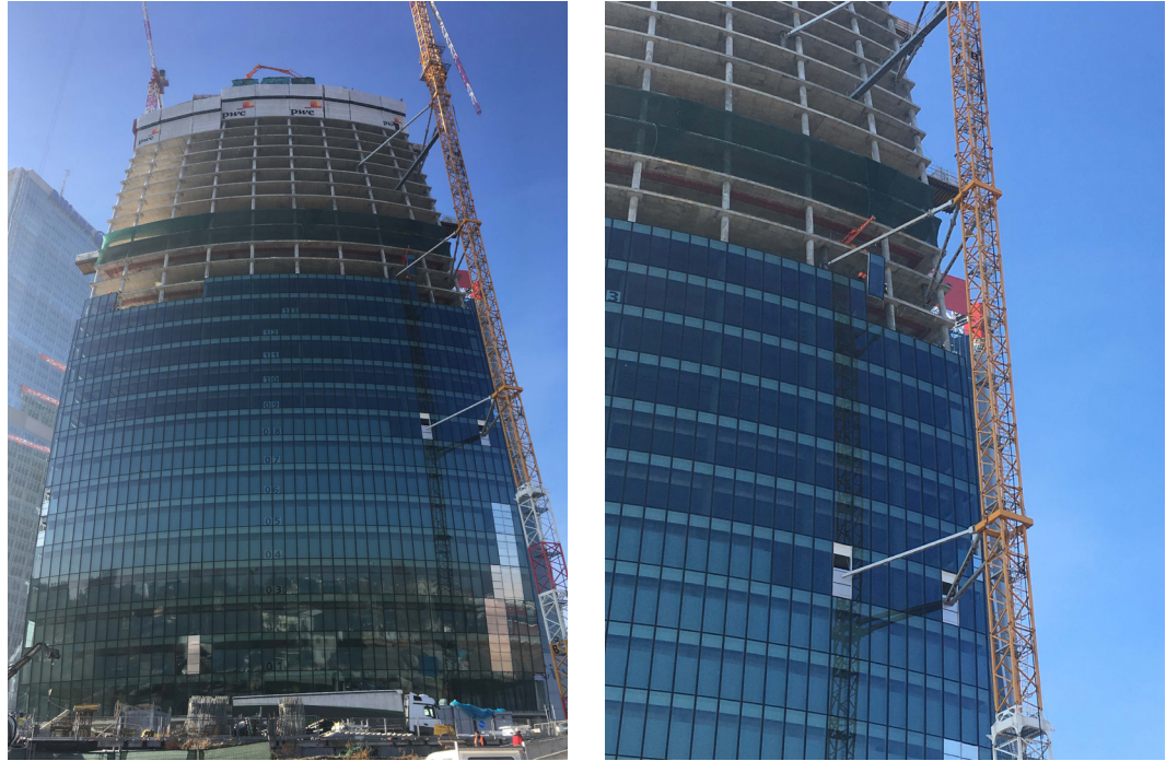
FIG. 7 Construction phases of the Libeskind tower façade
