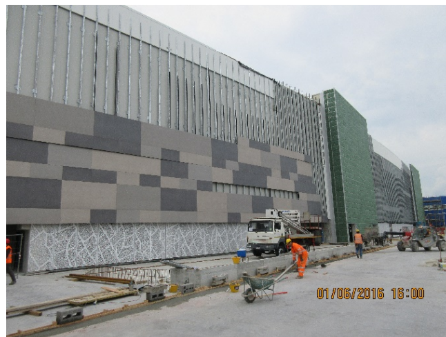
Fig. 3. During Construction (Living wall), Shopping Center, El Nos Roncadelle, Italy (source: authors)
