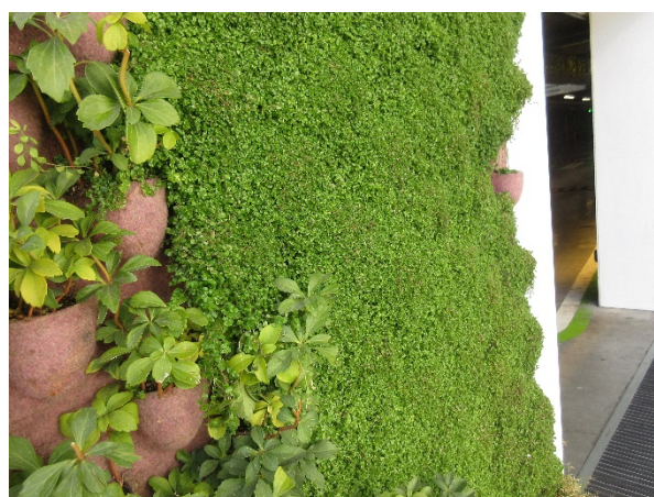
Fig. 7. Modular System, Shopping Center El Nos, Roncadelle, Italy (source: authors)
