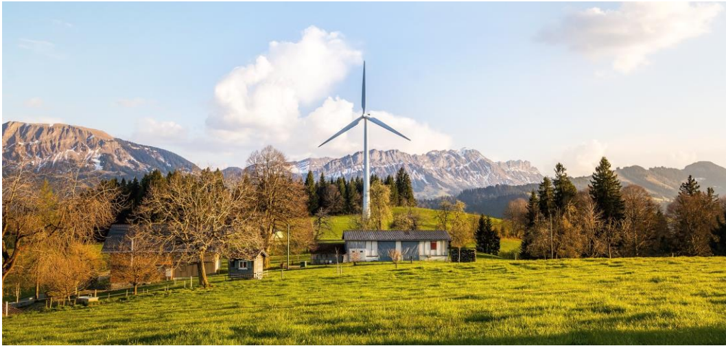
Figure 3 - Wind power plant in mountain area
