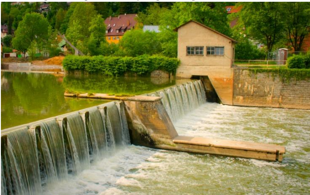
Figure 4 - Caption: micro hydro plant in agricultural area
