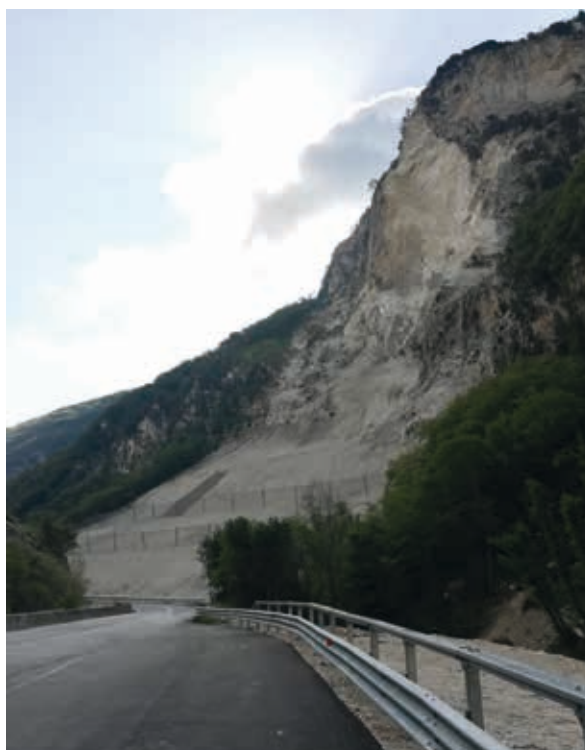
Fig. 5 - The SP 209 near Visso after the interventions (July 2018).
