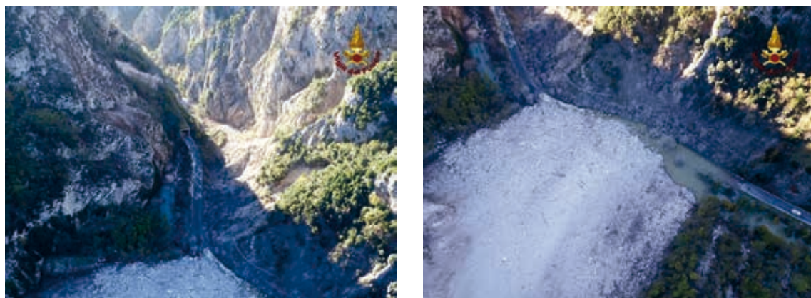
Fig. 3 - The rockfall triggered by the 30 October 2016 earthquake on the SP 209 and Nera River ( https://www.perugiaday.it/foto/cronaca/terremoto-norcia-frane-valnerina/aa644aa1.html#&gid=1&pid=1 ).
