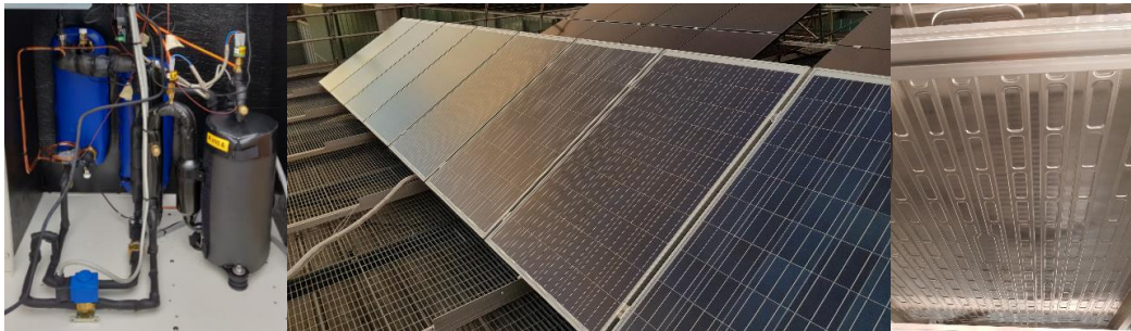
Figure 2 - From left to right: inside of the heat pump, front and back of PV/T modules
