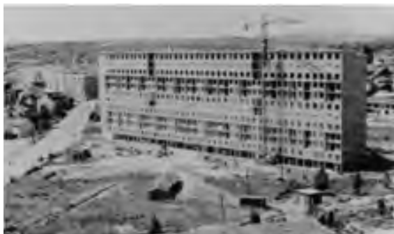
Figure 9 Construction of the peupleraié 1960
