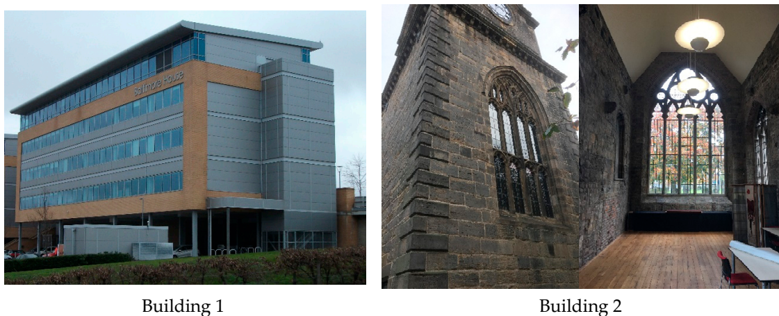
Figure 3. Images of Buildings 1 and 2 (source: field survey of buildings).
