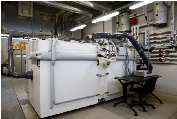
Figure 1: the DAVTB facility.
