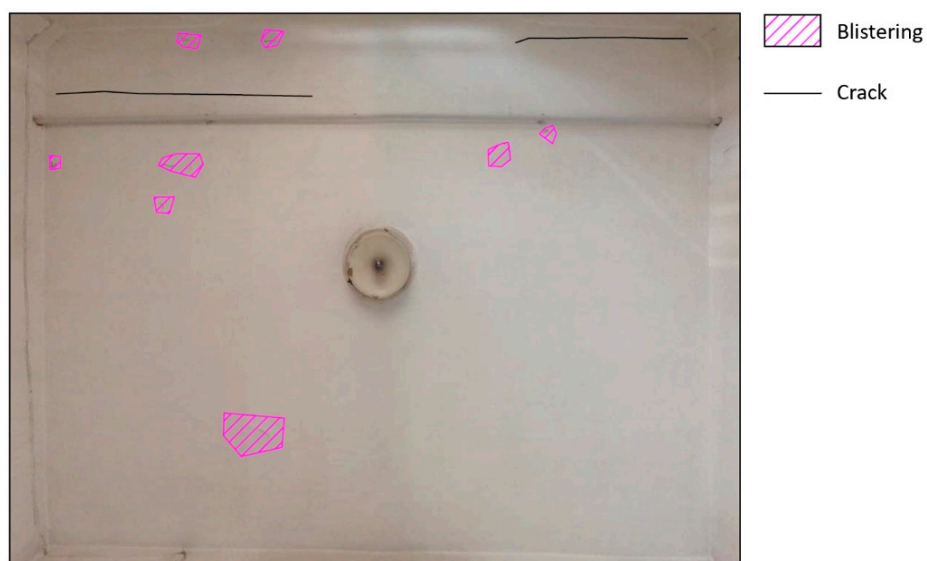
Figure 7. Results for the ceiling of the room. Areas were directly mapped on the rectified image to calculate areas and costs.
