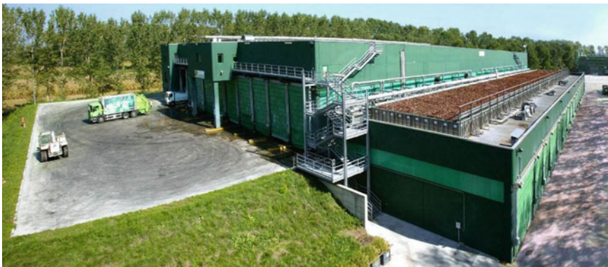
Fig. 2 View of a bio-drying system located in Italy, similar to the one described
