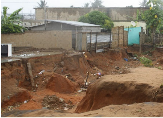
Fig. 3 Example of the harmful effects of uncontrolled urbanisation. Episodes of soil erosion due to torrential rains in a typical shanty town in the village of Maxixe (author's photos)
