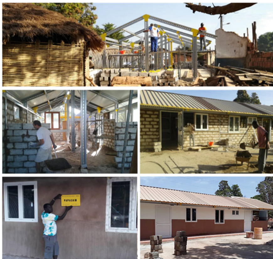
Fig. 11 Papagaio construction phases: structures earth block system and name plaque fixing
