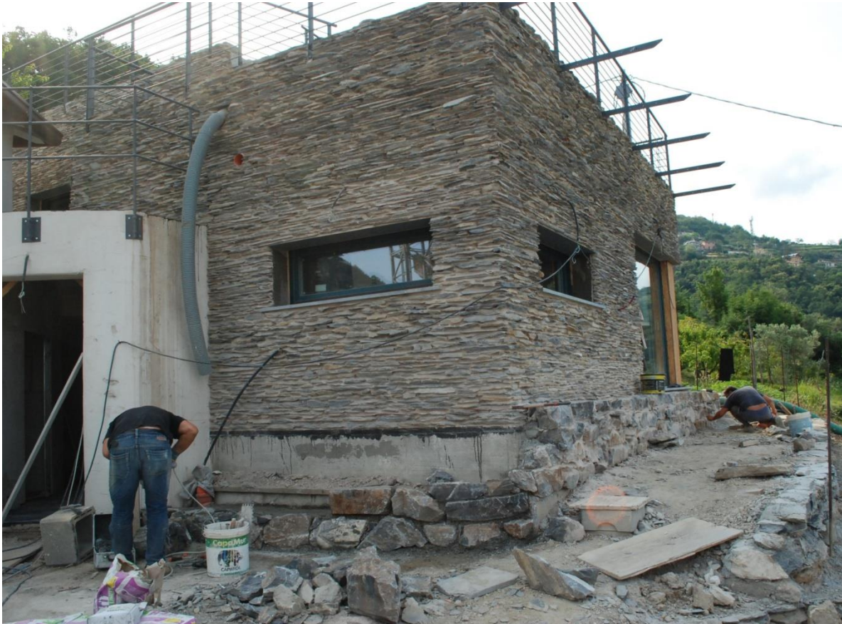
Figure 4. New body of “Villa degli ulivi” with external façade in local stones.
