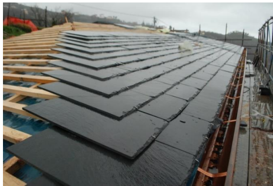
Figure 2. Detail of the roof with slate tiles.
