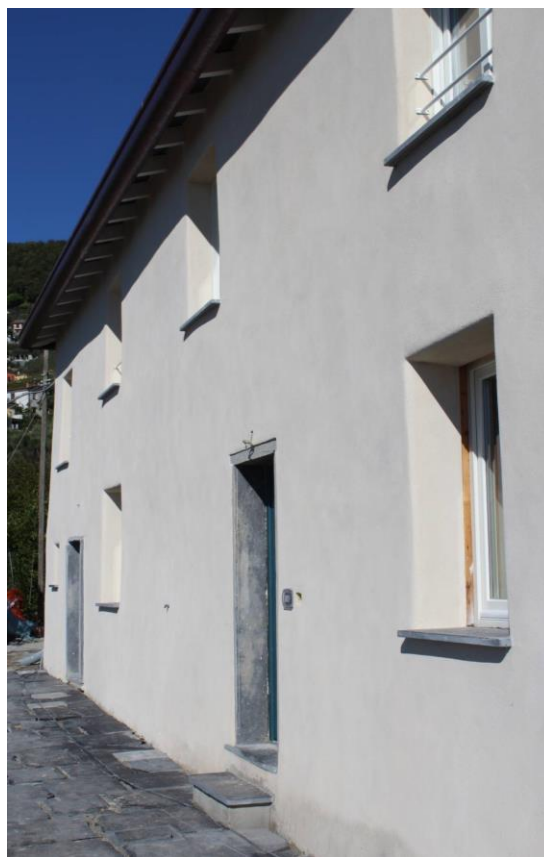
Figure 3. Part of the external façade with natural white lime mortar.
