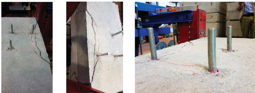
Figure 5. Specimen 3 after the shear test.
