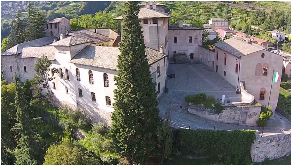
FIG. 2. Castel Masegra in Sondrio, Italy, surveyed with laser scanning and photogrammetric techniques for BIM generation.
