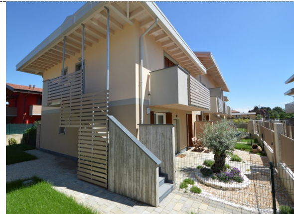
Figure 1. Building A, built with a load-bearing structural system of cross laminated timber.
