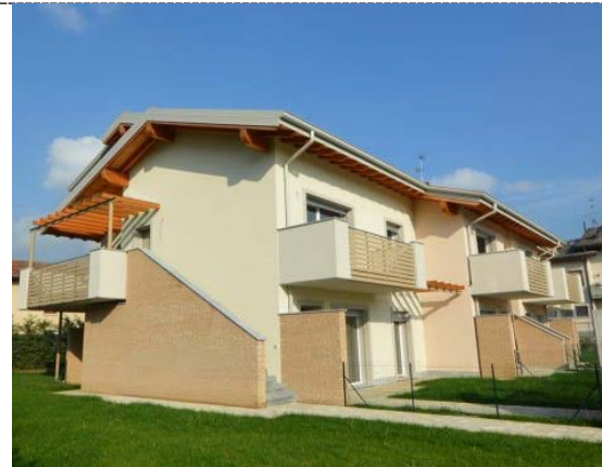
Figure 2. Building B, built with a reinforced concrete load-bearing frame and brick walls.
