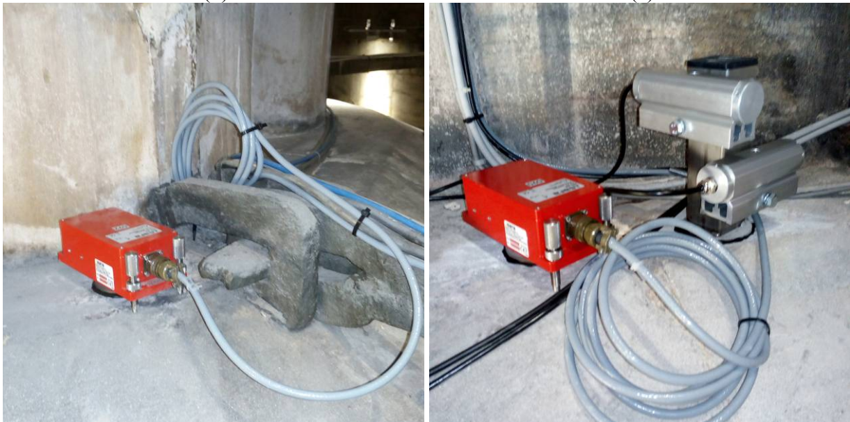
Fig. 7 Map (a) and views (b)-(c) of the seismometers installed inside the Milan Cathedral (dimensions in m)
