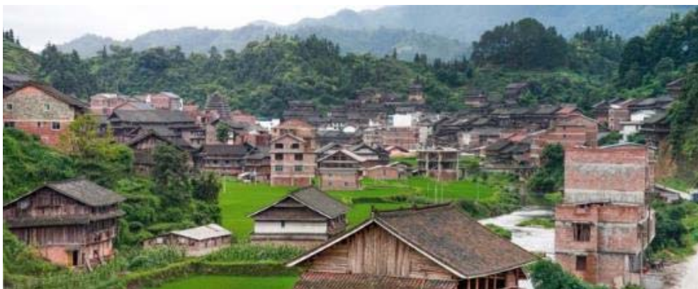
Figure 9. Construction chaos, Pingtan village (shot by Xiaotie Chen)
