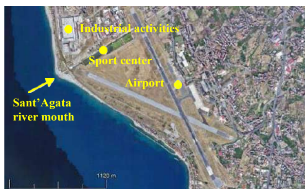
Figure 1. Detail of the final part of Sant'Agata river, it is possible to observe the airport, a sport center and industrial activities
