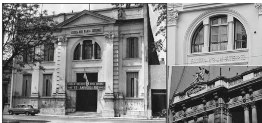
Fig. 10 Architectural elements composing the Morra's façade: tympanum, thermal window, pilasters in giant order, cornice
