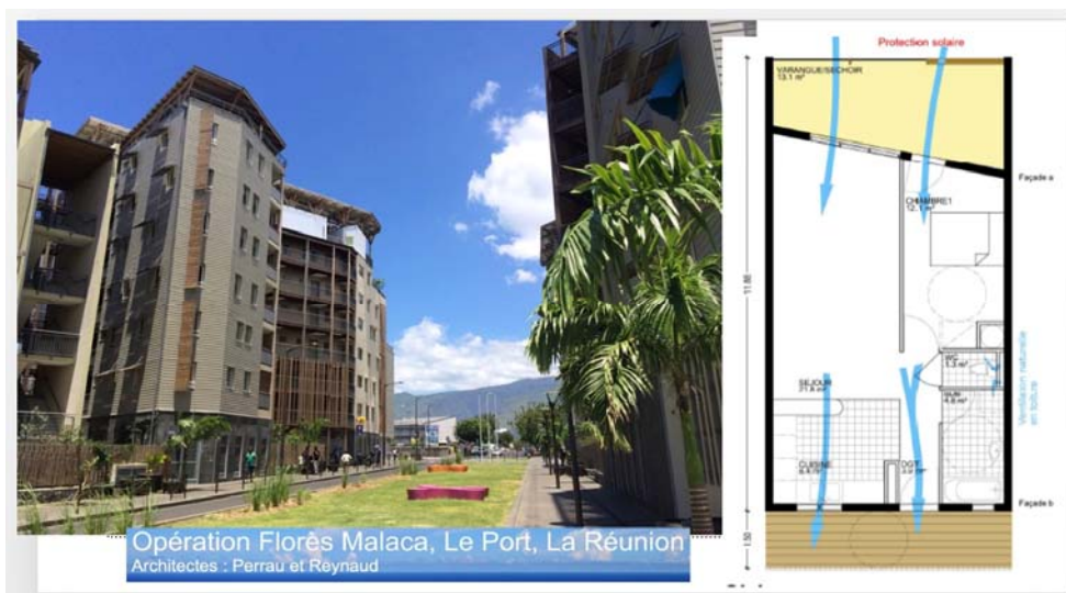
Figure 4. District of Florés Malaca, Le Port, La Réunion, and design of the apartments enabling effective cross ventilation
