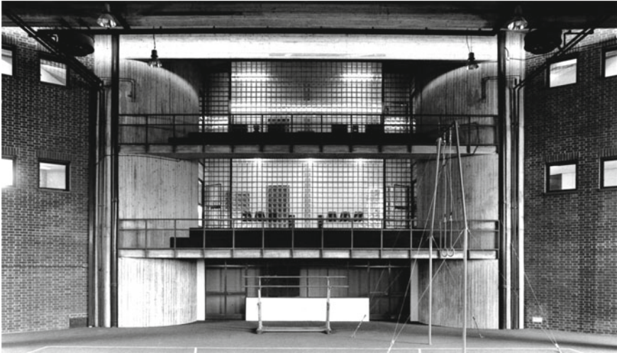
Fig. 5 Guido Canella, Civic Centre with a Town Hall, Middle School and Sports Field in Pieve Emanuele, Milan 1971
