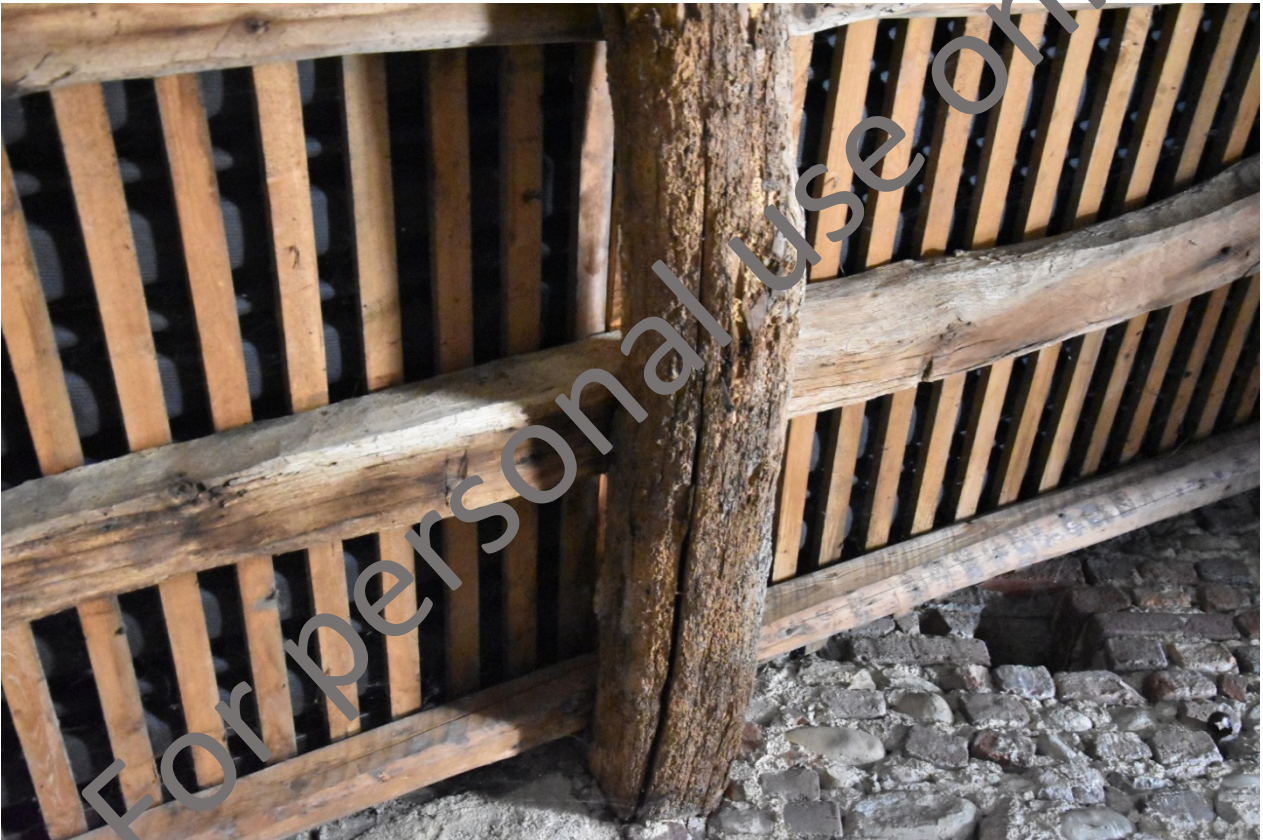
Figure 5. Biotic decay due to insects.
