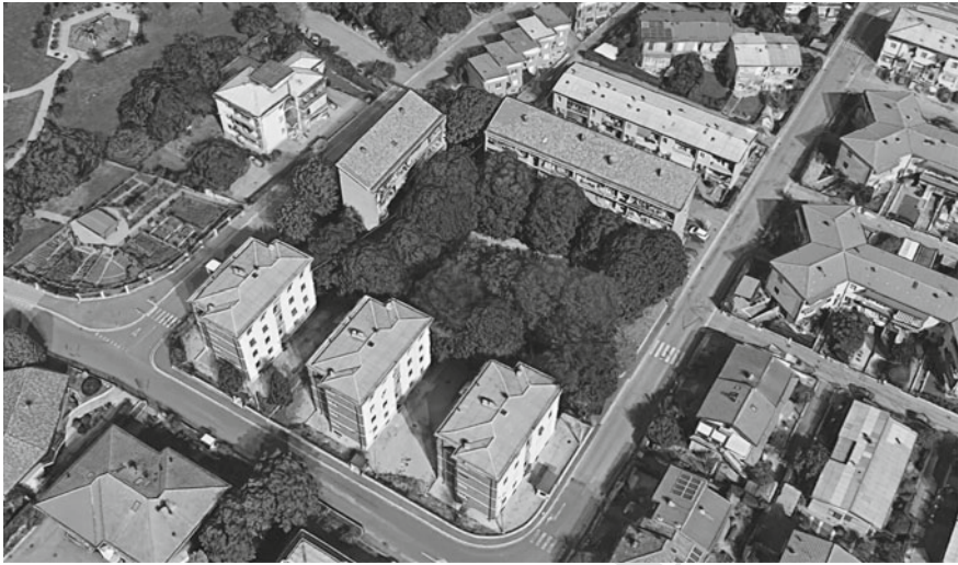
Fig. 1 Urban block of Piazzale Visconti with five buildings dedicated to public social housing. The three identical buildings are owned by the Municipality of Bergamo; the others belong to Aler
