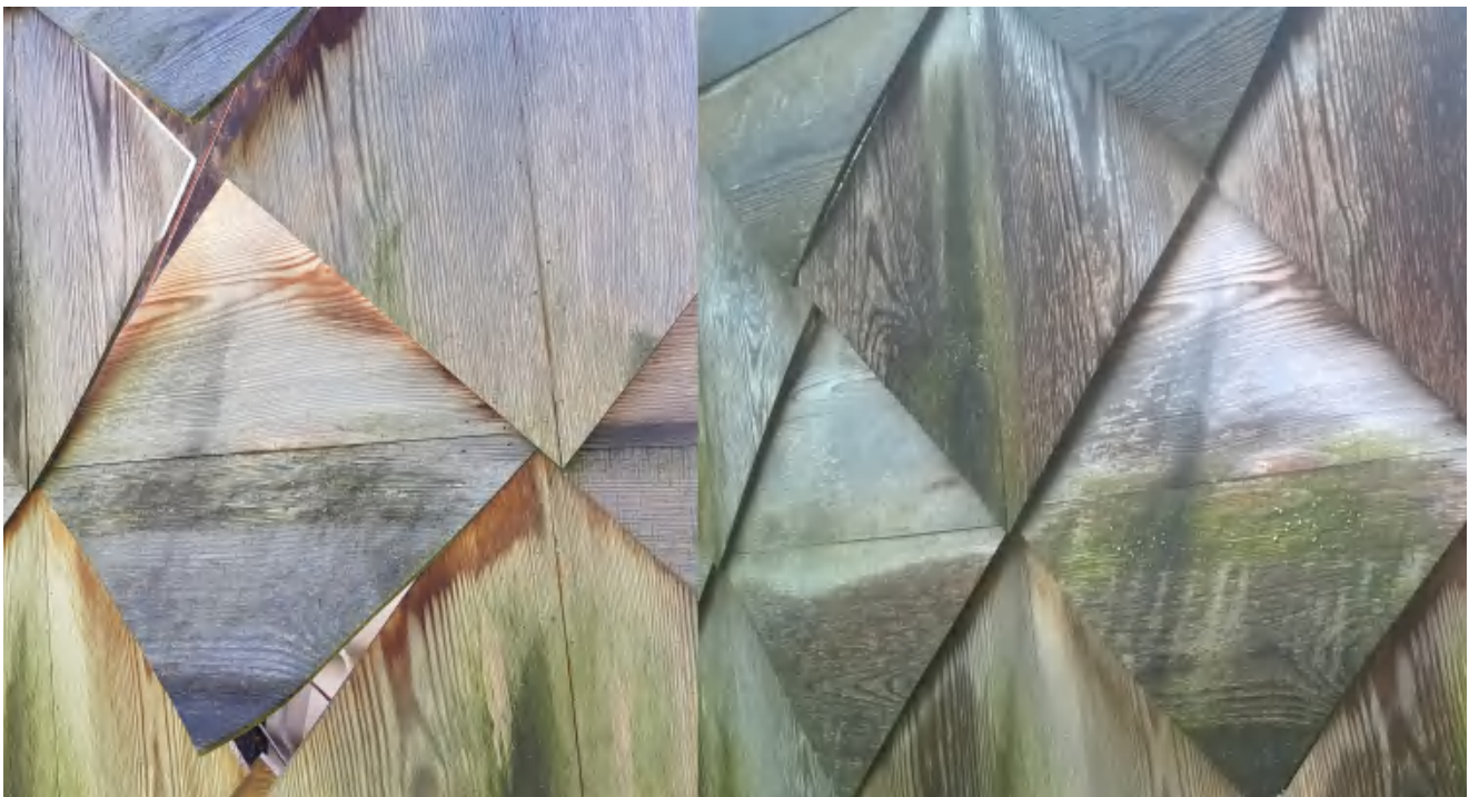
[Figure 2] Responsive solid wood screen Ray 2 co-performing with relative humidity, algae moisture sorption and temperature. The responsive wood panelling is moderating micro-climate: either producing humid air flow through its warping and moisture evaporation in hot and dry weather or sorping and enclosing it in humid and cold situation. This is moderated by algae moisture sorption: larger warping when dry and hot, prevention of warping in opposite direction when it rains. (photos: Davidová 2018 and 2017)
