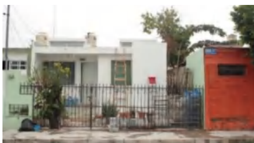
Image 6: Anahí Ramírez Ortíz Construction of ventilation for houses in Polígono 108
