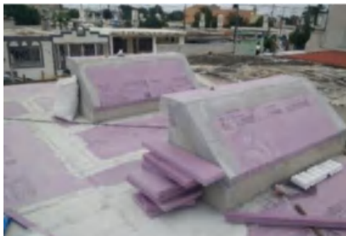
Image 5: Anahí Ramírez Ortíz NAMA Housing Retrofit Project, site visit, Polígono 108
