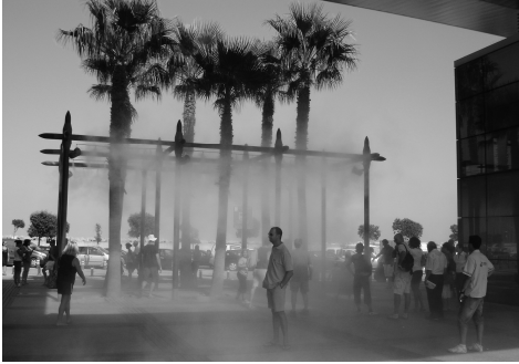
Fig. 4 - Cooling system with vaporisation at the Bastia seaport, Corse (source: photo by the author)
