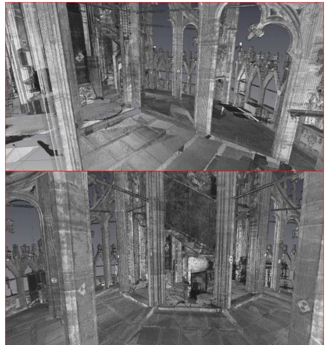
Figure 4. Some screen shots that show the registered point clouds of the dome cladding base.
