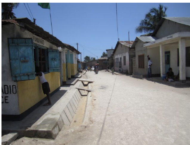
PHOTO 2 Stormwater drainage system, Tambukareli Ward
