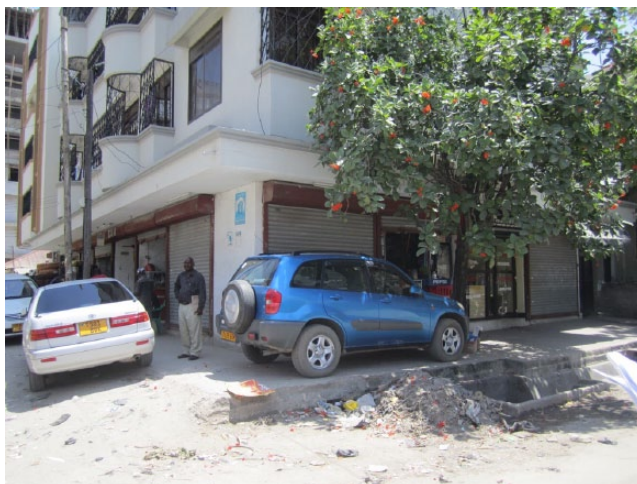
PHOTO 1 Storm water drainage system in Kariakoo
