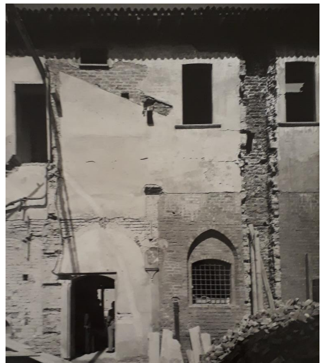
Figure 2. Space between the New Sacristy and the Cloister of the Prior, demolished after II World War to enlarge the New Sacristy and renew the layout of the complex.
