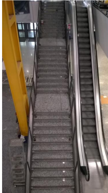
Figure 3: The staircase used for the experimental tests
