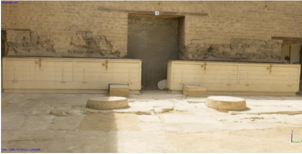
Figure 6. View of the 3D model of the tomb of Maya showing the wooden lockers located in the second courtyard, as surveyed (elaboration by F Fiorillo, 2018).
