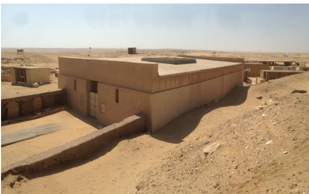
Figure 4. The tomb of Meryneith, encapsulated in a protective structure (photograph by L. Perfetti, 2019)
