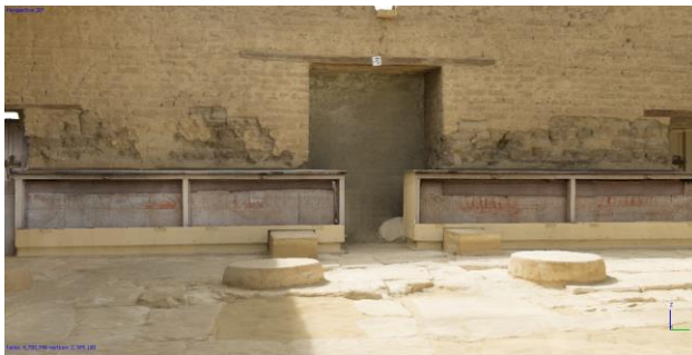
Figure 7. Same view of the 3D model of the tomb of Maya after the digital removal of the wooden lockers (elaboration by F. Fiorillo, 2018).
