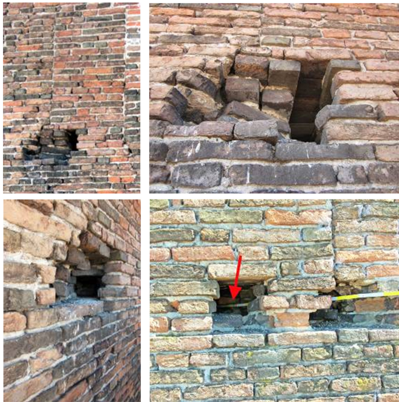
Fig. 6. Details of the infillings between the merlons on the N-W front.
